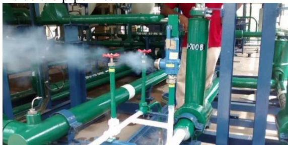
Fig. 4.5 Cryogenic pressure relief valve
