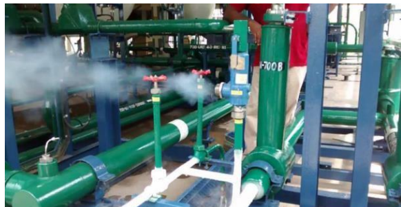
Fig. 2.1 Cryogenic PRV in operation at LSSF
