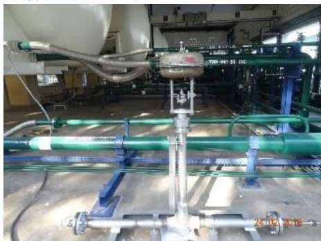
Fig. 4.3 Cryogenic globe valve
