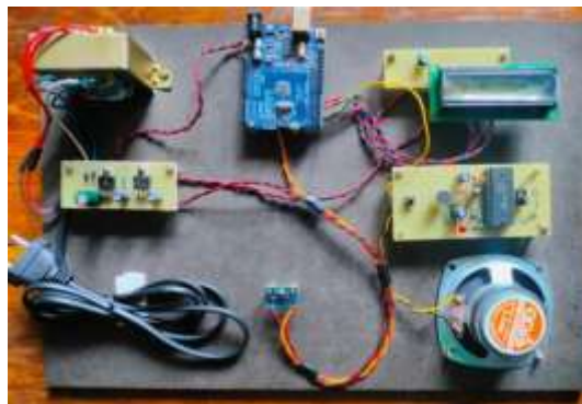
Figure 5: Earthquake detector without power supply
