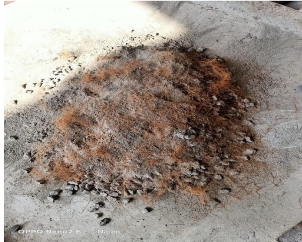
Fig. 12: Mixing of all ingredients for preparation of concrete.
