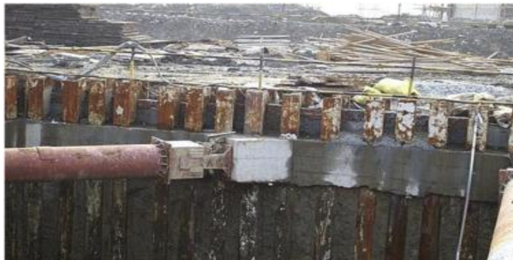
Figure 1. Constructed DSMW used in a subway project in Tianjin, China
