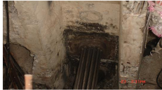
FIGURE (1) CASTING CONCRETE WITH GLASS FIBRE SURROUNDS PRESTRESS STRAND CABLE AT HOLAKAR BRIDGE
