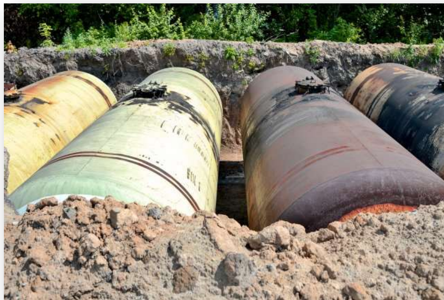
Fig 1. NAPL leak from the subterranean storage petrol station [4]
