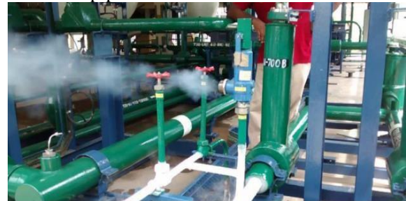
Fig. 4.5 Cryogenic pressure relief valve
