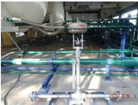
Fig. 4.3 Cryogenic globe valve
