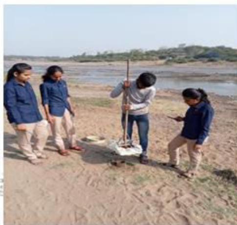
Fig 5 Setup of core cutter on site
